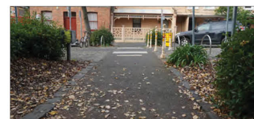
Raised pedestrian crossing with bluestone square sawn setts, tactile ground surface indicators and directional signage.
