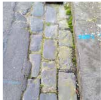
05 Three pitcher channel and bluestone kerb part of the site heritage fabric
