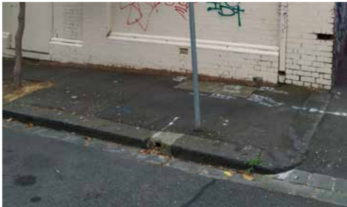
11 Typical existing footpath condition, bluestone kerb and pitcher channel
